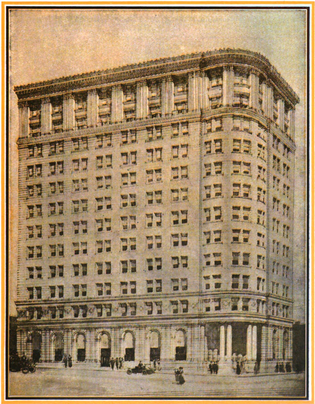
THE FIRST NATIONAL BANK, A STEEL FRAME STRUCTURE, WITH STONE FACING, FOR OFFICES, BANK AND SAFE DEPOSIT VAULTS; NORTHWEST CORNER MARKET AND POST STREETS, SITE OF THE OLD MASONIC TEMPLE; OWNERS, THOMAS MAGEE SONS COMPANY; COST, OVER $1,000,000; ARCHITECTS, D. H. BURNHAM AND COMPANY; DRAWINGS BY WILLIS FOLK
